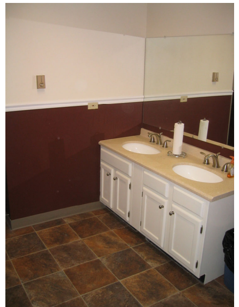
Erie Municipal Airport's newly remodeled bathroom
